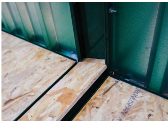
2.20 Place the wooden floor strip between the containers.
