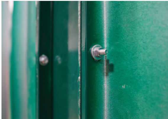
2.19 Secure side panels with M8 bolts.
